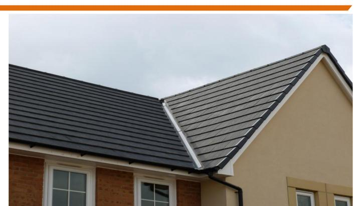
Polden is a thin leading edge riven finish flat interlocking roof tile which has the appearance of a slate when laid broken bonded.
